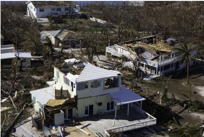
Figure 1: Damages in Treasure Cay/New Plymouth (Abaco) during an aerial reconnaissance flight
